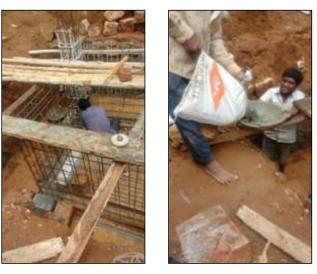
Fig 5 Portacrete<sup>™</sup> is being used for the column starters
