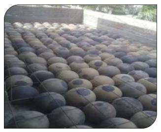
Fig 2 Ceramic pots placed in rows over the sunken slab
